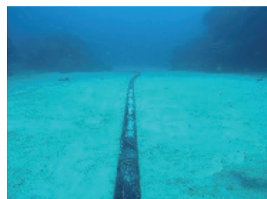
Laying submarine cables to avoid coral reefs
