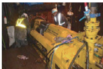
Workers burrowing below rivers to lay trunk line cables
