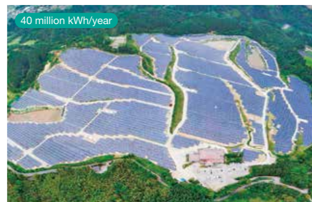
Miyazaki Kamenoko Solar Power Plant (Kunitomi Town, Higashi-morokata District, Miyazaki Prefecture)
