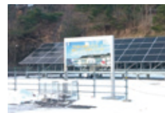
Hakodate Toi Building – Renewable-powered Telecom Facility
