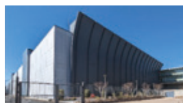
NTT DATA Mitaka Data Center EAST: The data center is scheduled to achieve virtually 100% renewable energy for its electricity use by FY2025 through the use of off-site PPAs and non-fossil certificates.
