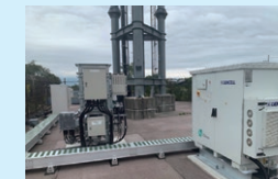
Equipment for a base station demonstration using hydrogen fuel cells
