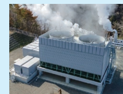
Geothermal power plant in Kumamoto Prefecture
