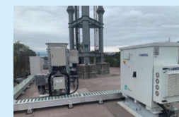
Equipment for a base station demonstration using hydrogen fuel cells
