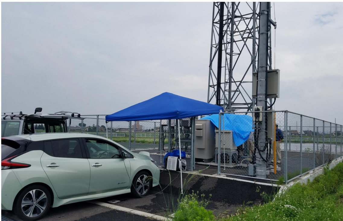
Fig. Image of the Demonstration Experiment (State of Power Connection between the EV and the Base Station)
