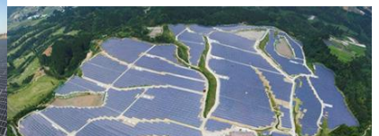
Miyazaki Kamenoko Solar Power Plant (Higashimorokata District, Miyazaki Prefecture) – 40m kWh/year –
