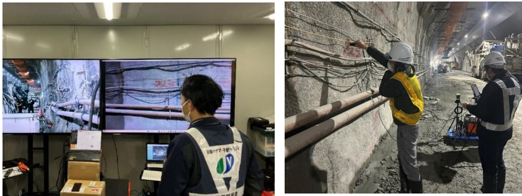
Photo 3. Remote Inspection Trial
