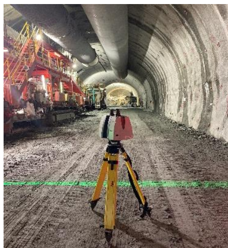
Photo 2. Point-Cloud Measurement Using a Laser Scanner
